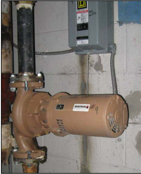
Heating Water Pump and Mixing Valve:
